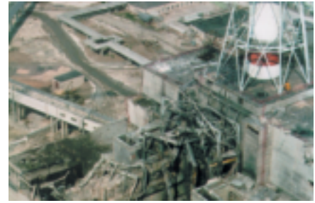
Fig. 2.36 The Chernobyl nuclear power plant following the accident in 1986.
