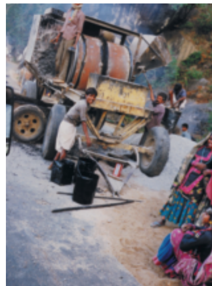
Fig. 2.19 Asphalt road-workers (shown here in India) are exposed to polycyclic aromatic hydrocarbons.
